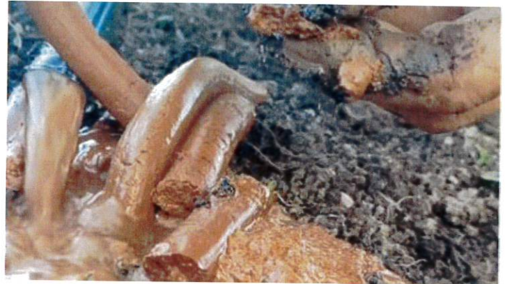
Clogged drip tape from unfiltered water
